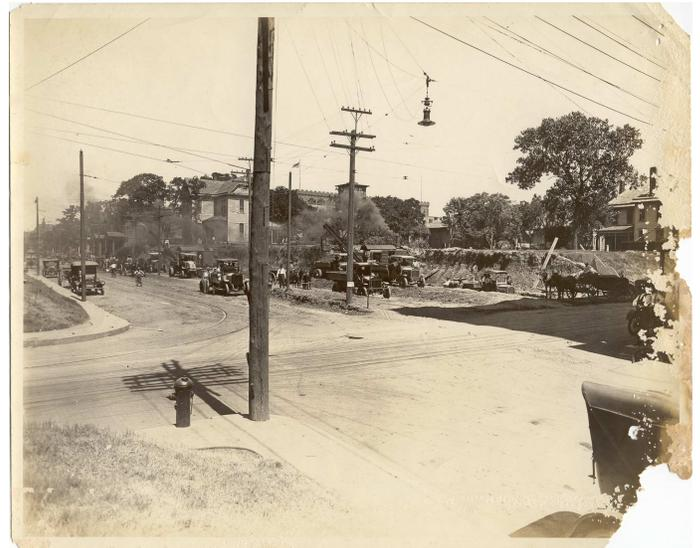
“Vilbig Bros. have secured a nice contract for excavating the basement of the new Federal Reserve Bank Building at Dallas. There are about 25,000 cubic yards of material to be moved on this contract. They have two small revolving shovels on the job, loading the dirt into Western Dump wagons and trucks.” excerpt from *The Earth Mover: A Monthly Magazine for Earth and Stone Movers*, Volumes 6-7, March 1919 Number 1.
